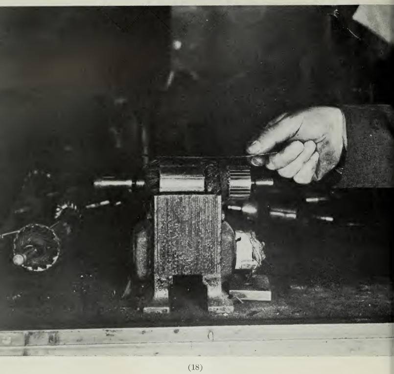
The armature is tested for shorts. This is done by placing the armature onto a magnetic growler (that is, by setting the core part on the magnet) and if there is a short in the armature, a thin metal blade will be attracted to the core, as shown above.
